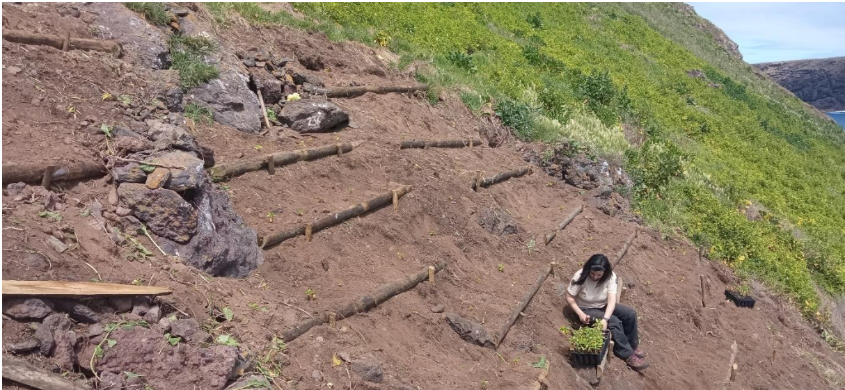
Figure 10. Wooden palisade construction and planting in areas of IAS removal on Vila Islet, Santa Maria, in April 2023.
